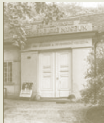
12 | Entrance and gate of building No. 97 in the lower part of Kinsky Gardens in Prague-Smíchov.
